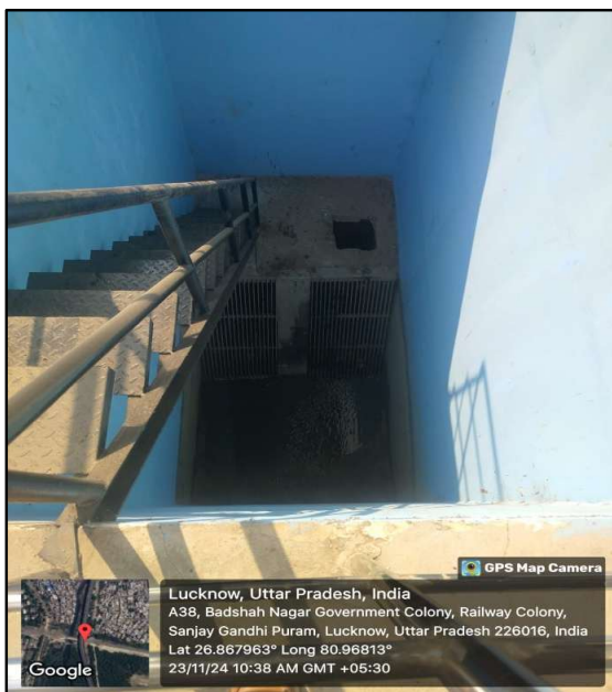
Badshah Nagar, Pumping Station Mesh Filtration
